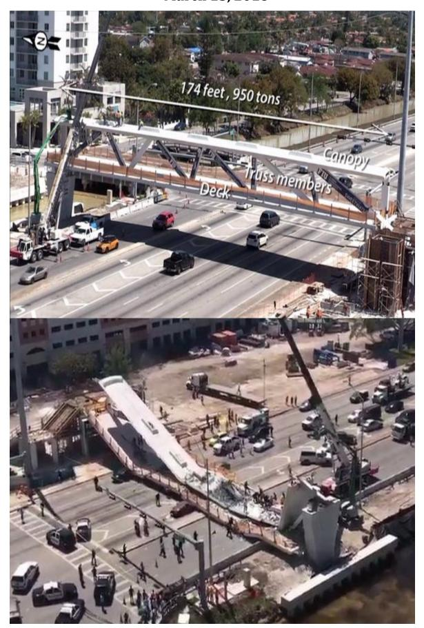
On March 15, 2018, a 175-foot-long (53 m) structure that was a section of a pedestrian bridge that was under construction at the FIU campus near Miami, Florida, collapsed onto the road below (Tamiami Trail). This incident resulted in six deaths (5 motorists and 1 employee), eight injuries, and eight vehicles being crushed underneath.
